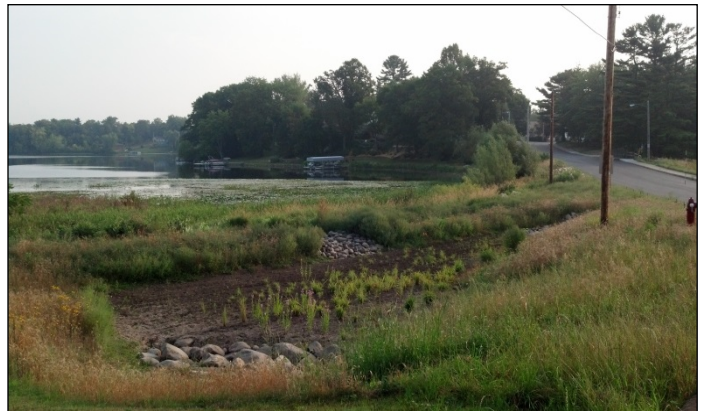
Stormwater runoff is treated by a recently constructed stormwater treatment pond, pictured above, before entering Library Lake. Photo Credit: EOR, Inc.
